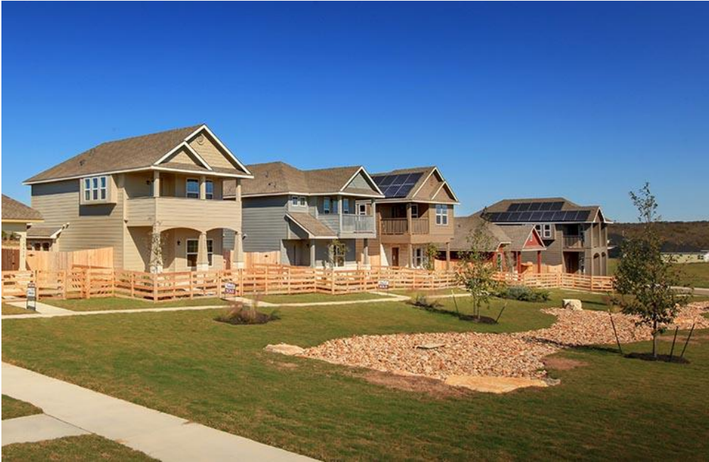
Francis Solar was contracted to install a rooftop solar array on every home in the Whisper Valley development. Upon completion, the total solar output will be an estimated 37.5 MW. Whisper Valley
